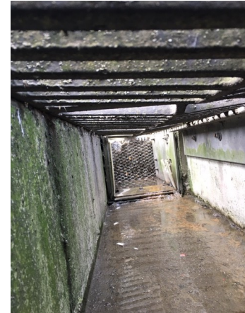
Trench drain after filter, all clean!
